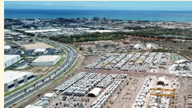
Industrial / HART Yard
